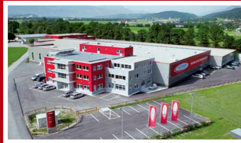
Heliotherm Heat Pump Competence Center 2.260 m 2 office space , 3.100 m 2 production area, 3.250 m 2 warehouse space
